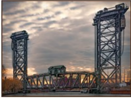
.AW~Vertical Lift Bridge~Jack Martin
